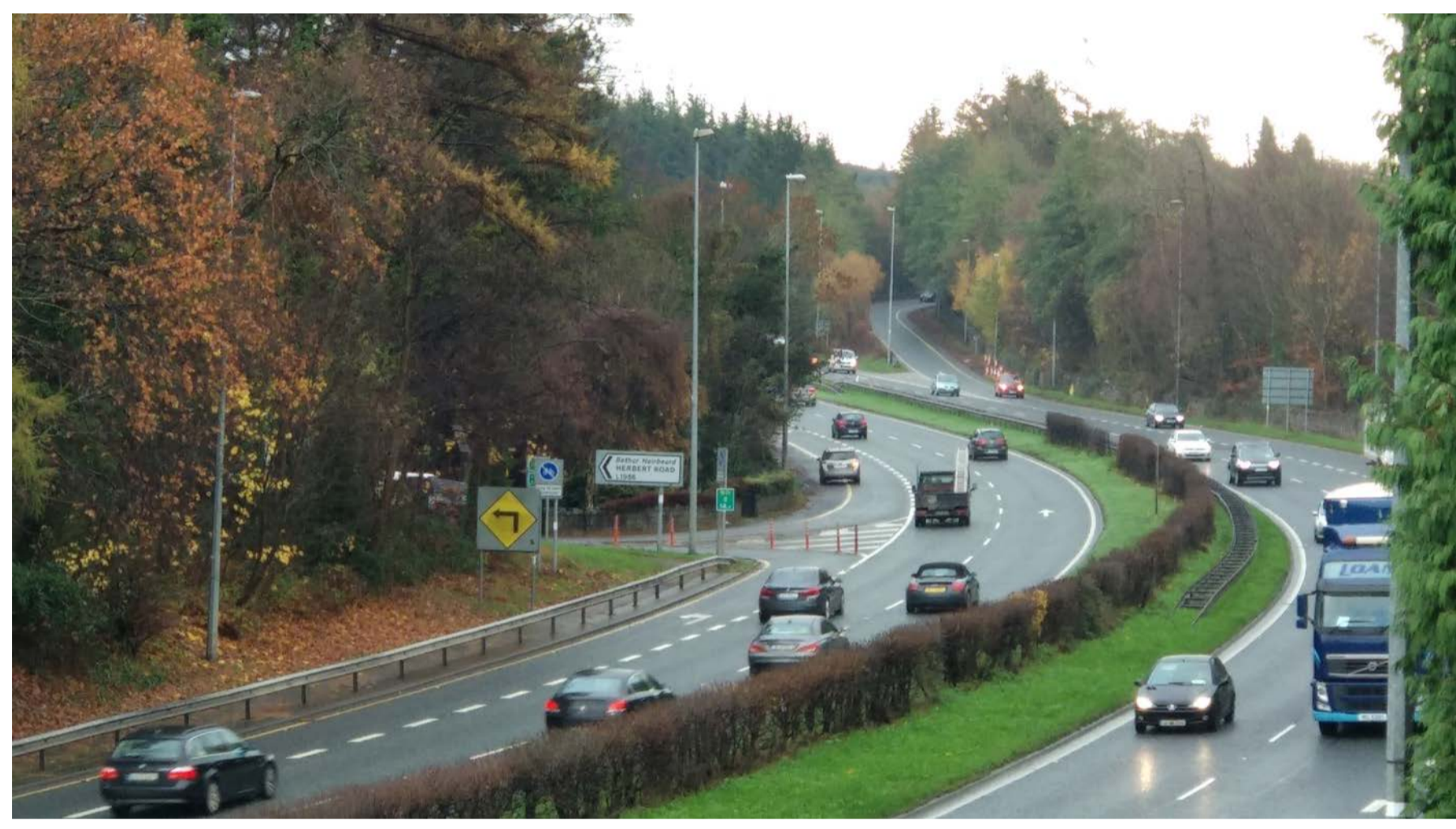
R117 Enniskerry Junction
