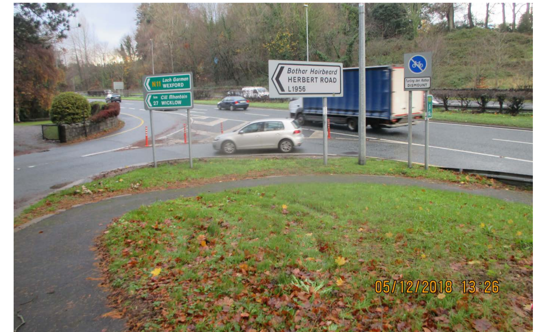
Herbert Road Junction
